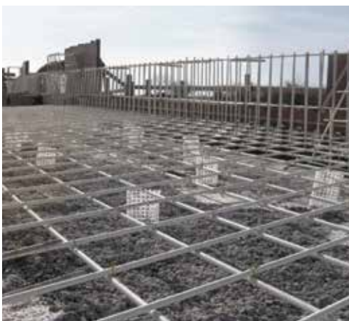
Reinforcement of the bridge cap of the Canal Bridge, Canada
