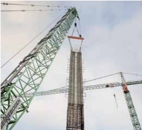
2nd S-Bahn main line, Munich, Germany (©Moritz Bernouilly)
