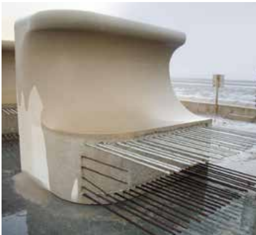
Precast elements along the beach promenade in Blackpool, UK
