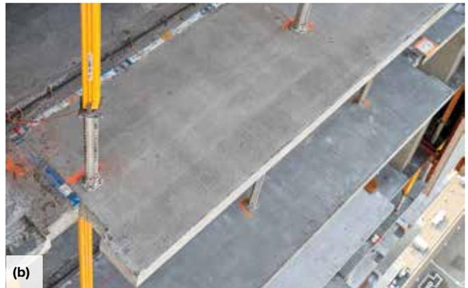
Fig. 3: Structural thermal breaks in balconies: (a) during placement of balcony concrete; and (b) after placement of balcony and slab concrete. Note: Modules are installed with the top plate flush with the exterior concrete structure. The white bars are GFRP bars
