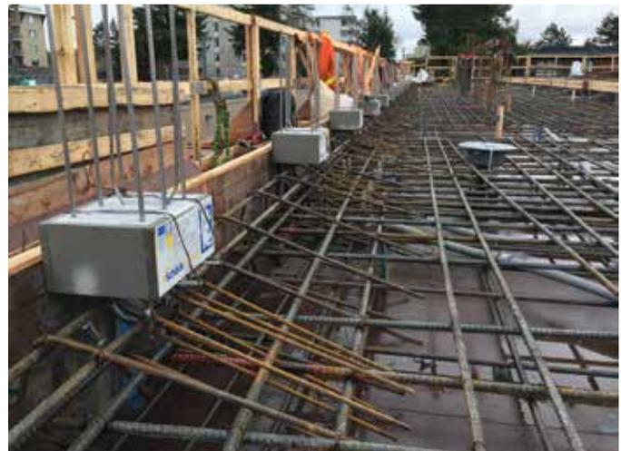
Fig. 4: Thermal breaks for parapets are installed at the vertical wooden parapet forms and tied into the horizontal reinforcing bars. Reinforcing bars are fabricated to transfer both bending and shear across the insulation layer
