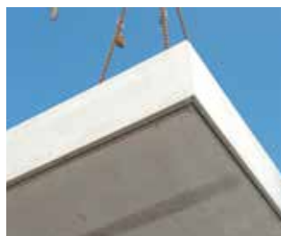
4. Remove the sealing strip after the element is lifted
