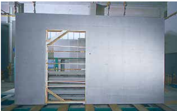
Conventional wood formwork
