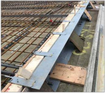
Fig. 20: Use of a continuous steel jig
