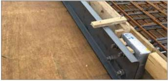
Fig. 19: Use of a continuous steel jig
