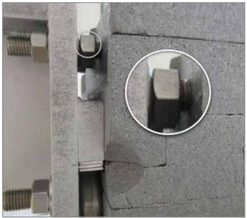
Fig. 31: Inner nut on the upper bolts for the adjustment of a camber
