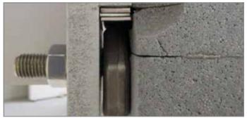
Fig. 27: Placing of the steel construction using the shims on the product to overcome vertical tolerances
