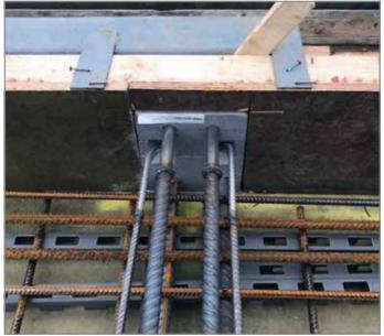
Fig. 17: Opening in slab edge formwork with integrated Schöck Isokorb® type KS and installation jig behind
