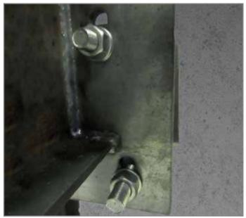
Fig. 28: Vertical slots to allow for vertical tolerances up to 20 mm
