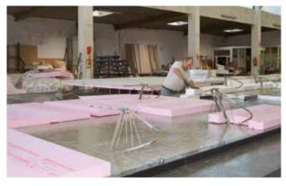
${\bf 1.}\ {\bf Cover}\ {\bf the}\ {\bf freshly}\ {\bf cast}\ {\bf concrete}\ {\bf outer}\ {\bf leaf}\ {\bf with}\ {\bf thermal}\ {\bf insulation}$
