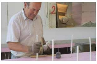
2. Insert the Thermoanker into holes drilled into the thermal insulation  $% \left( 1\right) =\left( 1\right) \left( 1\right) \left$
