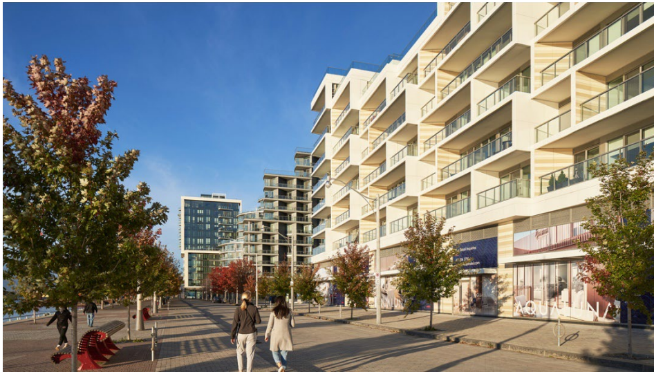
Balconies are insulated with Isokorb® structural thermal breaks to prevent thermal bridging.
