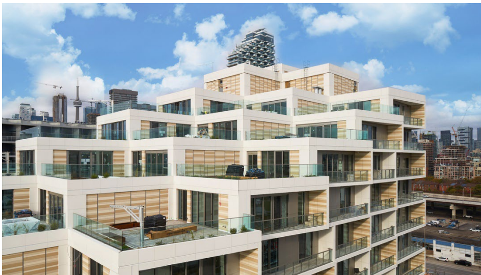
Exterior of the completed Aquabella condominiums depict layered architectural design and extensive balconies which are insulated with Isokorb® structural thermal breaks.
