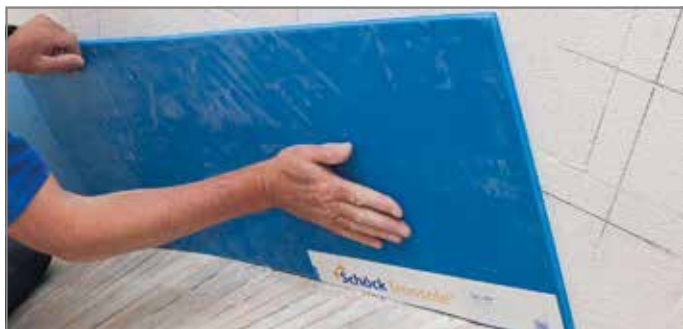
Ill. 131: Coller le Tronsole® type L
