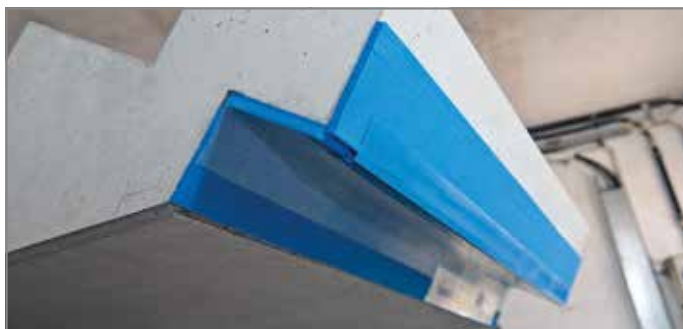
Ill. 109: Tronsole® type BZ installé
