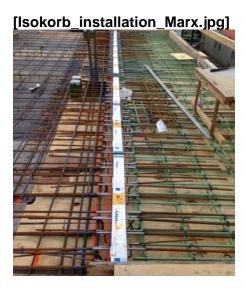
Installation of Schöck Isokorb® type CM structural thermal break for concrete balcony and slab connections in the Marx, Astoria Gardens.
