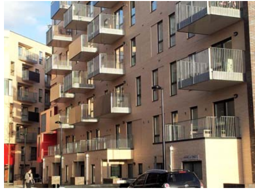
A recently completed phase
