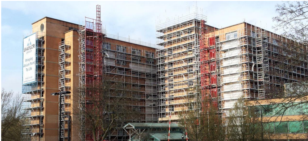
Work in progress at Sudbury Hill. Image: Schöck Ltd.
