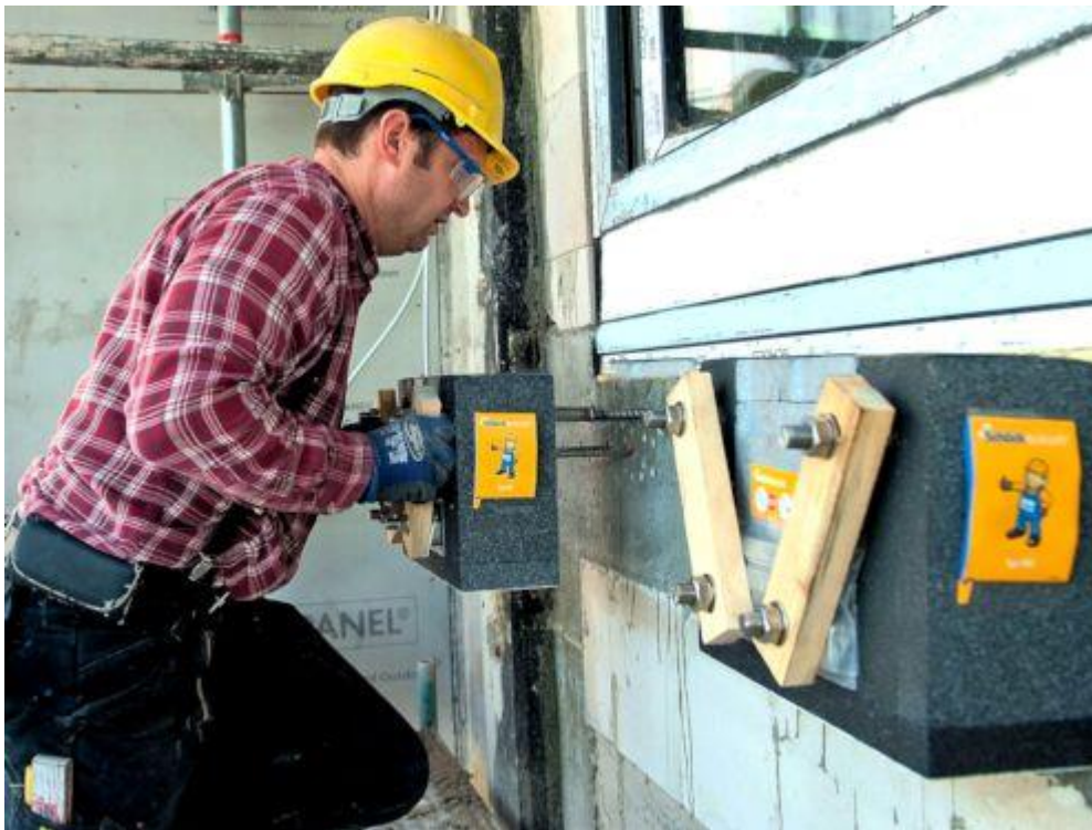
General example of the RKS being installed. Image: Schöck Ltd.
