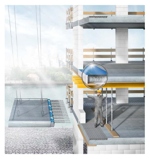
The new Schöck Isokorb ID for retrofitting balcony slabs during the structural building phase.
