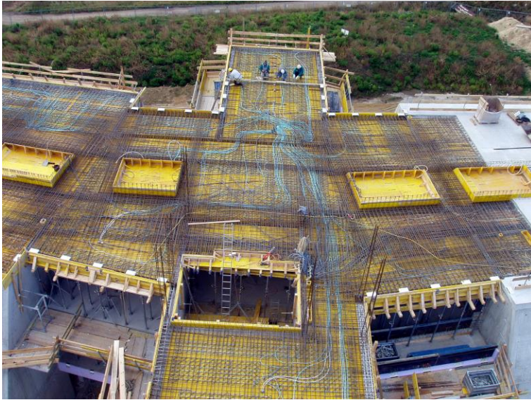
Early site work at the Velux Headquarters.
