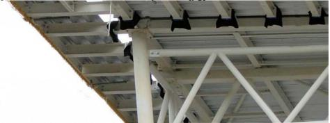
The structural elements to the primary steel are isolated from the interior environment using Isokorb structural thermal break units from Schöck. The Isokorb is one of the most sophisticated solutions on the market, for the prevention of thermal bridging in connective situations.
