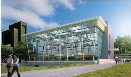
The New Stillhouse – When complete, Midleton will be one of the most modern distilleries in the world. The 21.5 m high pot still hall building envelope is designed to a very high level of thermal performance and one of the design factors that had to be taken into account was the prevention of thermal bridging.
