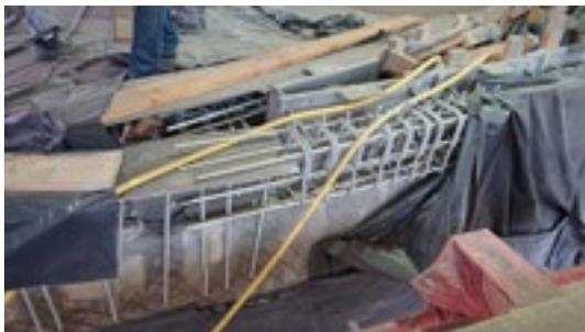
*Edge beams were formed in the roof area of the TWIST. Schöck Combar reinforcement cages also guarantee reliable load transfer here.
