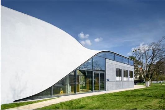
*The CUBE in Dresden, the world's first carbon concrete building, was constructed entirely without steel reinforcement.*
