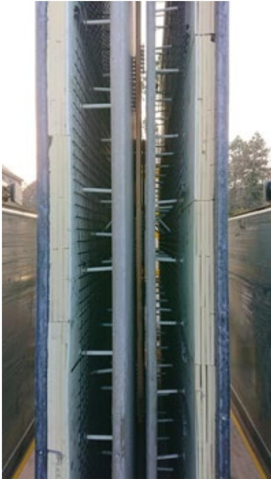
*The structure of the composite walls is clearly visible here. The cavity is filled on site with in-situ concrete.
