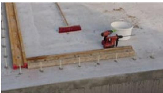
*Schöck Combar is used as connection reinforcement in the foundation of the BOX, and absorbs the load of the external walls.*
