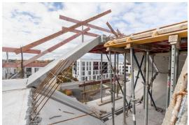
The honeycombs consist of horizontal in-situ concrete slabs and inclined hybrid precast elements. Photo: Edward Beierle
