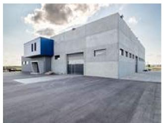
The high-quality concrete facade featuring the natural stone look of the new precast plant was made possible thanks to the use of Schöck Isolink. Photo: Schöck Bauteile GmbH
