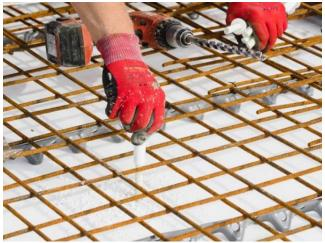
The Schöck Isolink Type C-SH for the attached outer shell panel is set into the insulation at a depth of at least 6 cm. Photo: Schöck Bauteile GmbH
