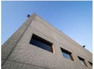
Façade elements with a load-bearing shell panel made of concrete (15 cm), insulation made of expanded polystyrene (12 cm), and an outer shell panel (8 cm). Photo: Schöck Bauteile GmbH
