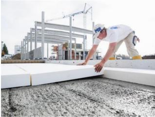
The insulation layer made of expanded polystyrene (ESP) comes after the outer shell panel with the concrete. Photo: Schöck Bauteile GmbH
