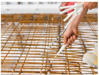
The Schöck Isolink Type C-SD for freely suspended outer shell panels is set into the insulation at a 45-degree angle. Photo: Schöck Bauteile GmbH
