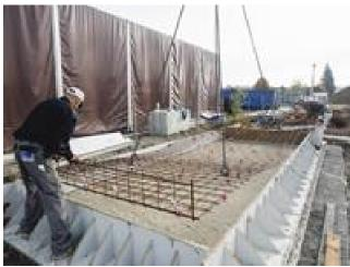
Installing the reinforcement elements on the outer shell panel. Photo: Schöck Bauteile GmbH
