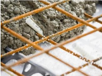
The load-bearing shell panel is concreted as the last layer. Photo: Schöck Bauteile GmbH
