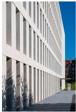
*Every façade component was sandblasted at the precast plant. Photo: Schöck Bauteile GmbH*
