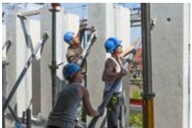
The façade is made up of more than 350 precast concrete components, with variously designed individual elements with two to four shafts. Photo: Schöck Bauteile GmbH
