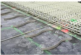
Laying the spacers for compliance with the concrete cover. Photo: Moritz Bernoully
