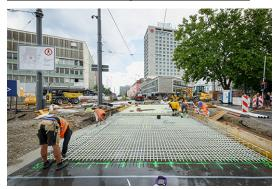
*The "lower layer" of the reinforcement immediately before completion. Photo: Moritz Bernoully*
