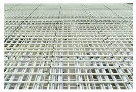
View of a floor slab reinforced with Combar. Photo: Moritz Bernoully
