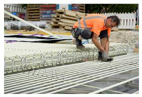
Fixing the reinforcement with cable ties. Photo: Moritz Bernoully
