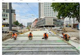
Work on the "lower layer" of the reinforcement. Photo: Moritz Bernoully
