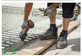
The Combar reinforcing bars are cut to the correct length. Photo: Moritz Bernoully
