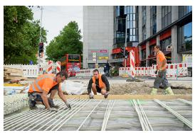
Align the longitudinal bars according to the spacing prescribed in the reinforcement plan. Photo: Moritz Bernoully
