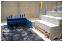
The Tronsole is installed directly on site before the assembly of the staircases. Photo: Schöck Bauteile GmbH
