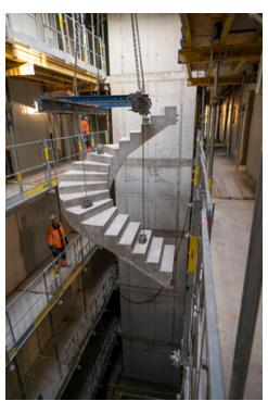
The half-spiral stair flights of the "immergrün" project were produced as precast elements. Photo: Schöck Bauteile GmbH
