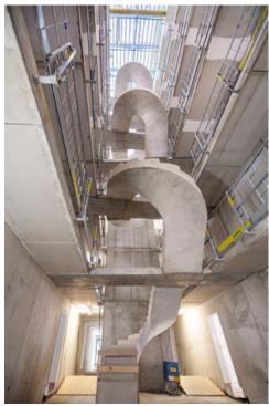
Walkways span the outer walls of the atrium, which can be reached from the galleries. The central, hanging, half-spiraled reinforced concrete staircase provides access to each floor via the walkways. Photo: Schöck Bauteile GmbH
