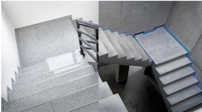
*As long as the blue line is continuous and unbroken, the component is successfully acoustically insulated from other structural elements. Schöck Bauteile GmbH*
