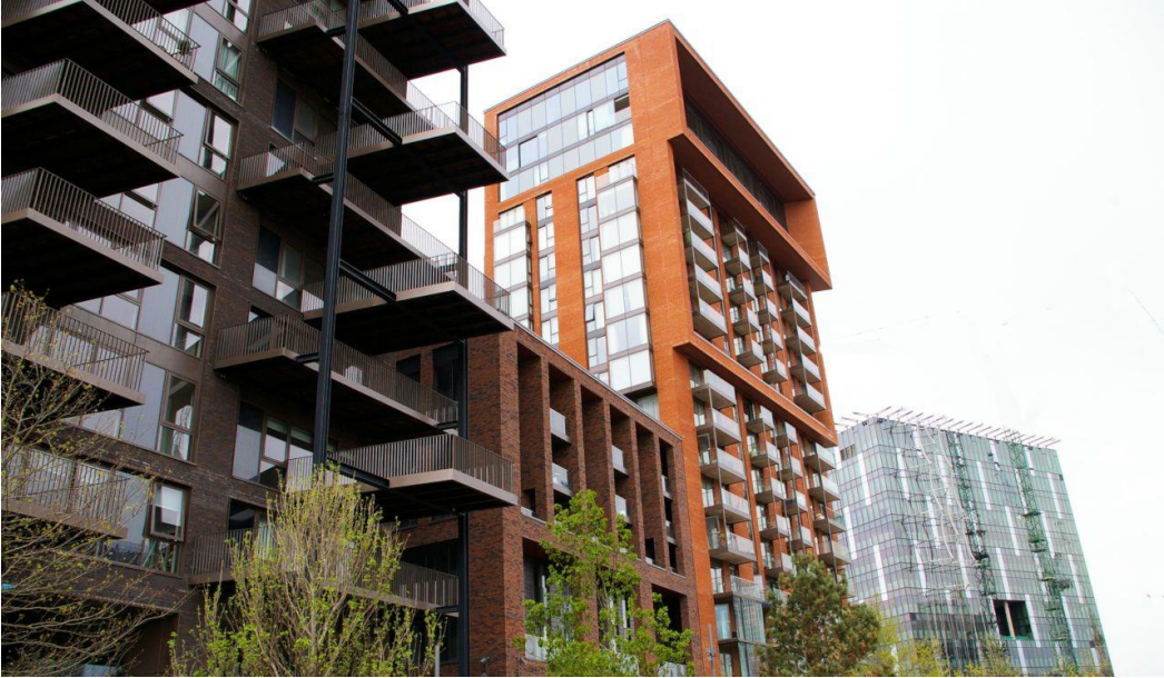
The rear of the development with the new US Embassy under construction in the background
