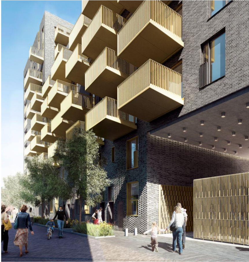
The main entrance area with the large balconies clearly evident Image: Project Orange
