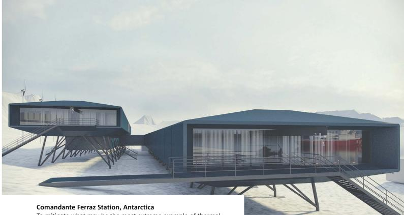
To mitigate what may be the most extreme example of thermal bridging in the world, the project team deployed 218 Schock Isokorb<sup>®</sup> structural thermal breaks between the building's interior steel-framing and its exterior steel support pillars and staircases. Architect: Estúdio 41, Brazil
