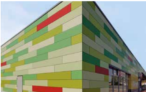
Example of a rainscreen cladding façade: REWE Markt, Laatzen © AS Hibbeln GmbH
