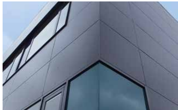
Example of a rainscreen cladding façade: Training Centre, Niedersachswerfen © Dach Schneider Weimar GmbH
