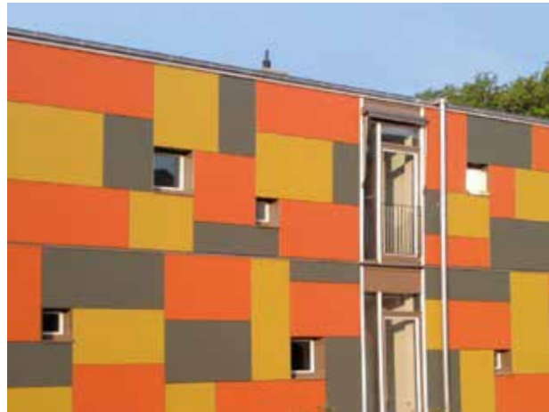
Example of a rainscreen cladding curtain façade: St. Konrad childcare centre, Burghausen © AS Fassaden GmbH
