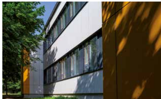
Schöck reference: School, Osnabrück © Schöck Bauteile GmbH
