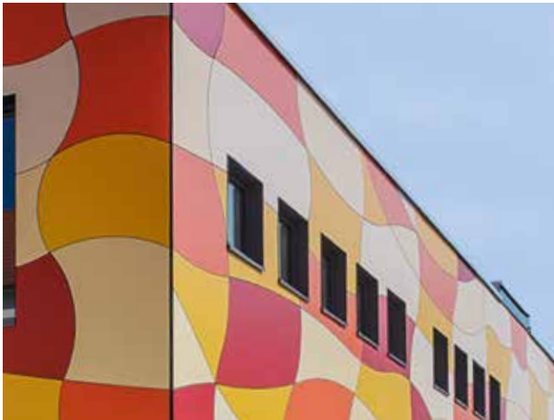
Example of a rainscreen cladding façade: Grammar school, Hoyerswerda © bauhoys Planungsbüro
